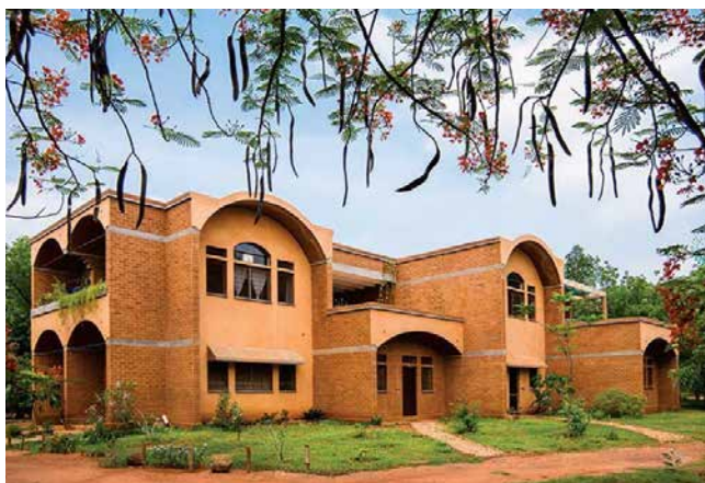
A community building in Auroville, India using compressed stabilized earth blocks
